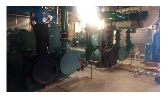
50,000,000 ton-hours of cooling by supplying 42° F water used to cool and dehumidify air entering and circulating in the buildings. Chilled water consumption is metered at each building on the distribution system. In 2022, Emory nearly completed construction to upgrade chillers in the Michael Street chiller plant that will significantly boost reliability and efficiency for meeting the campus cooling load.
