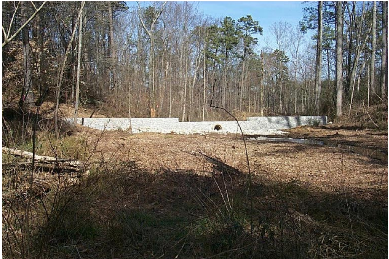
Figure 3d Starvine Way detention dam looking toward silt pond.
