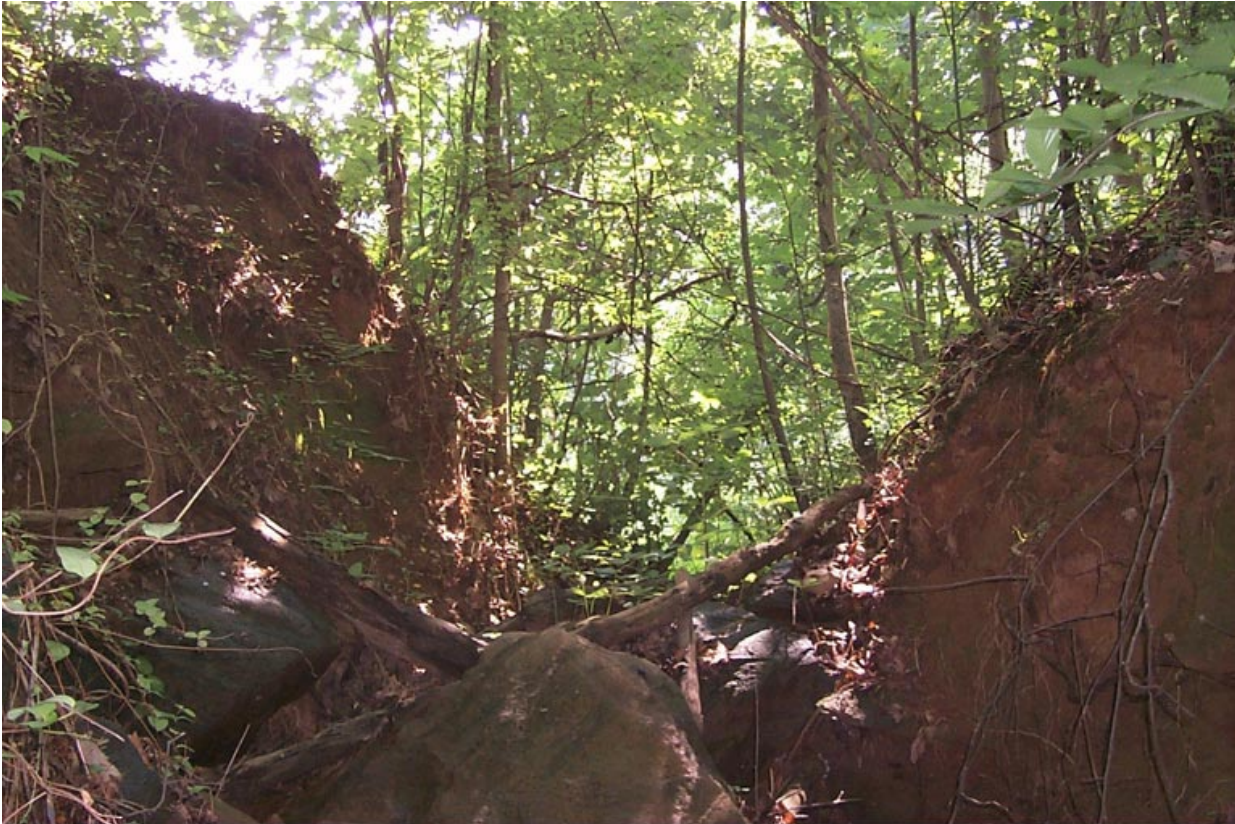
Figure 3b Breach in spoils dam.
